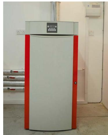
the fuel is critical to efficient biomass boiler operation, so a dry pellet storage area is required.
